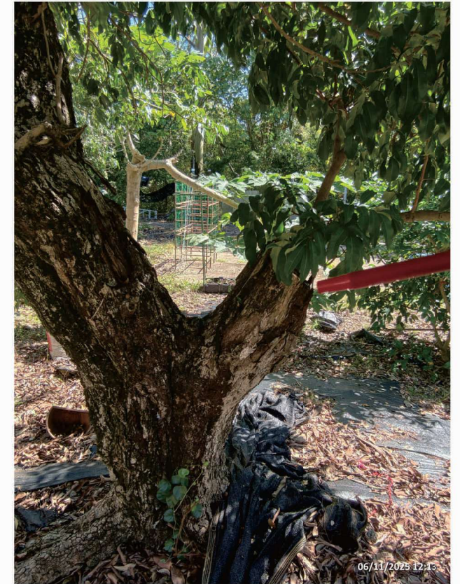
B10 (F) - Decay Stub in Trunk
