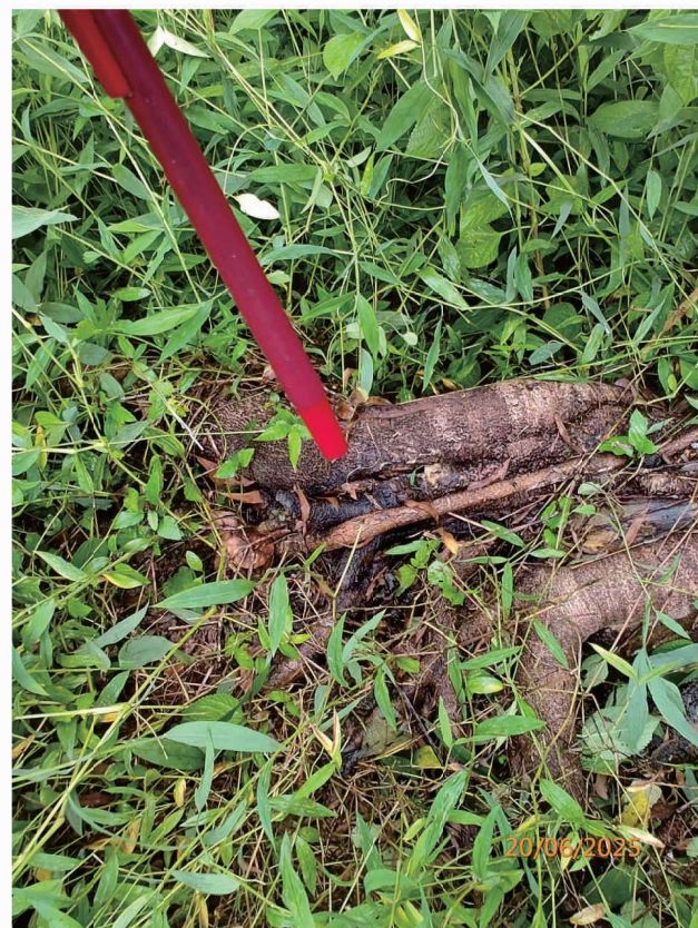
A02 - Decay in Trunk Base (F)
